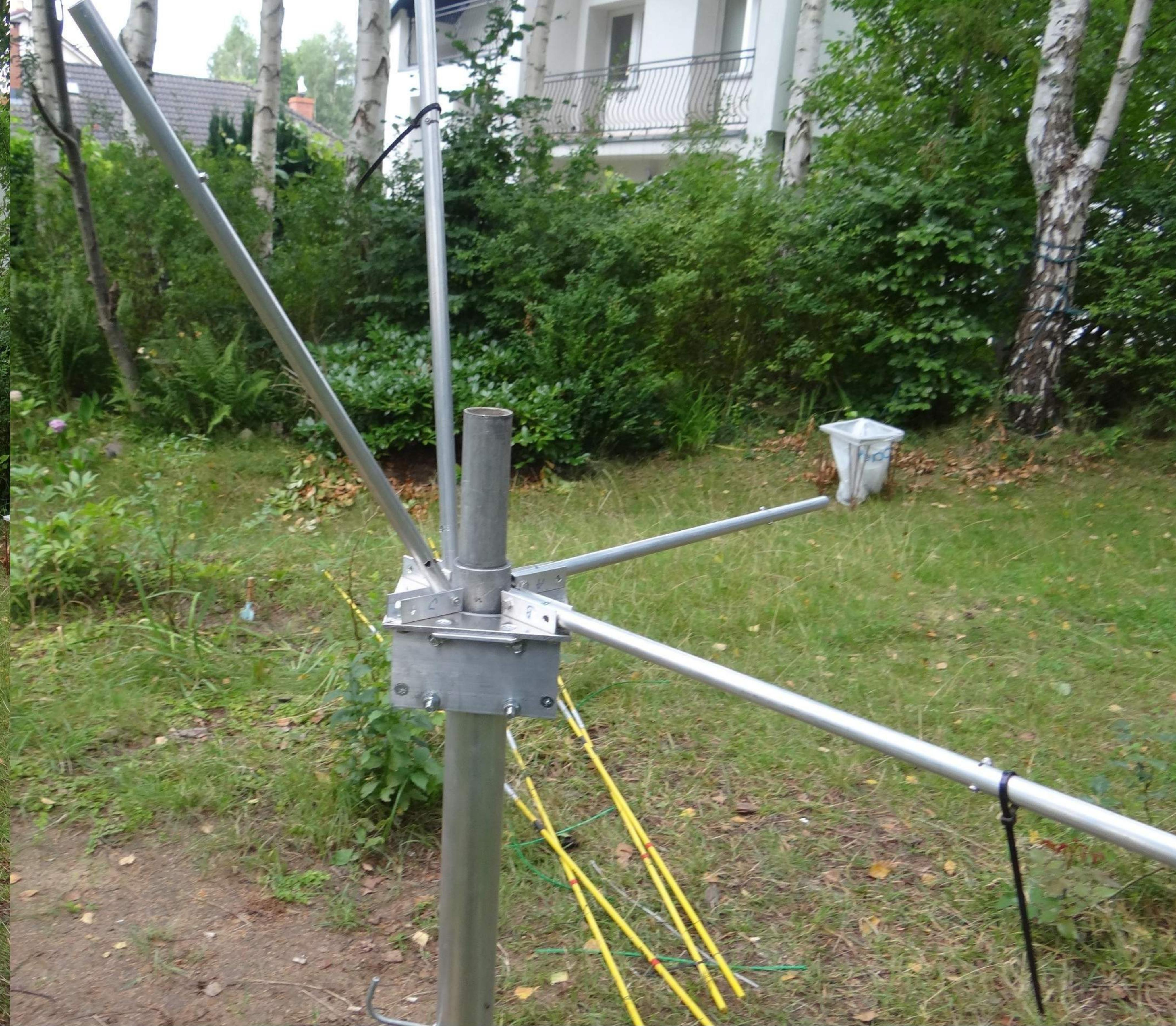
First, install the aluminium crossbar on the mast (at the end of the mast, maximum diameter 50 mm), leaving at least 120 cm clearance from the top to install the rope holder supporting the antenna arms.
