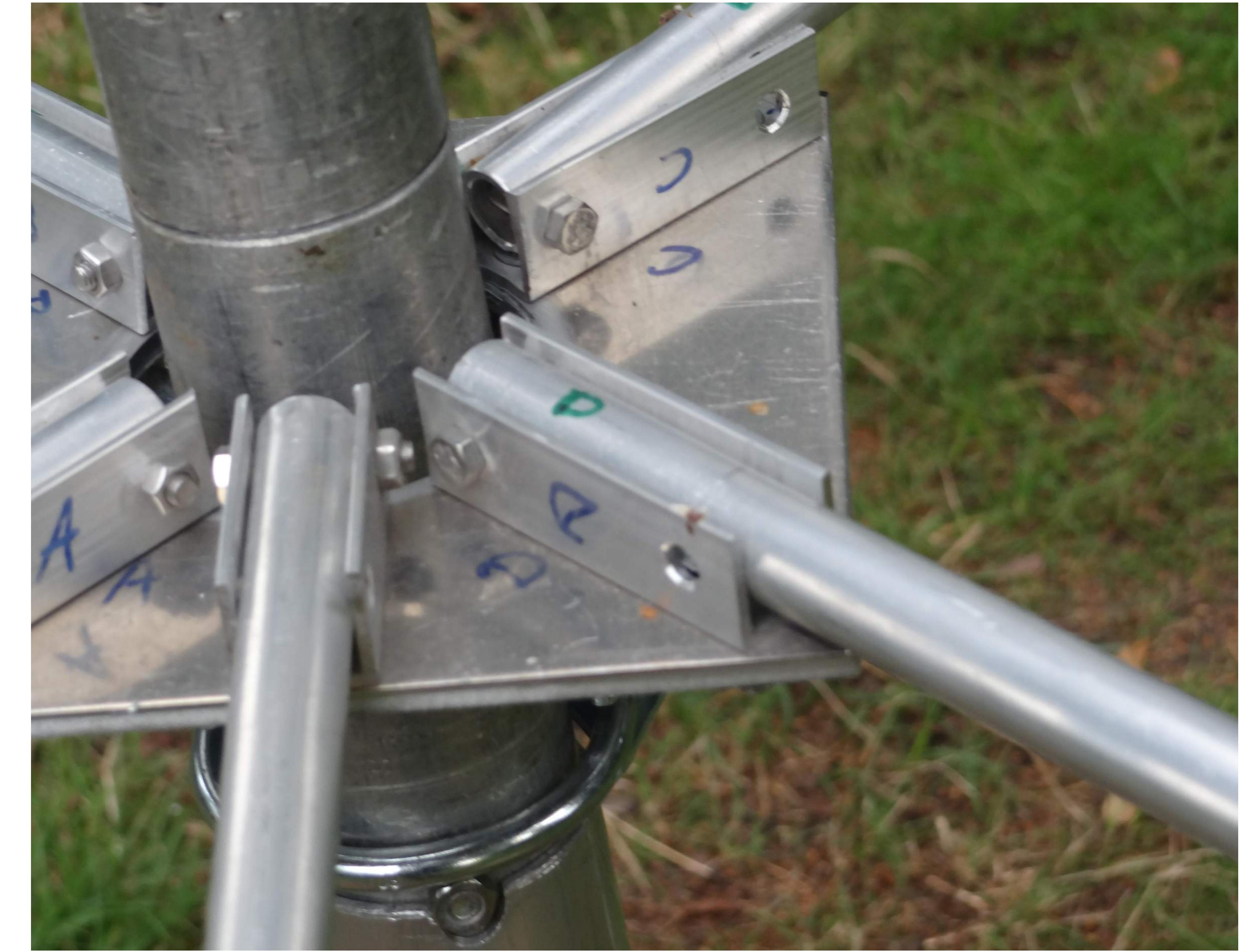
We can see the 50 mm diameter mast passing through the head hole and the arm sequence marking.
